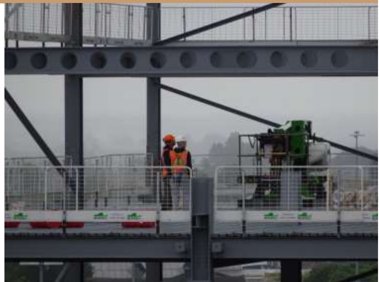
📍 Council offices at Friargate under construction
